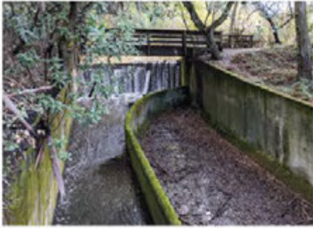
1 EXISTING DAM INFRASTRUCTURE
