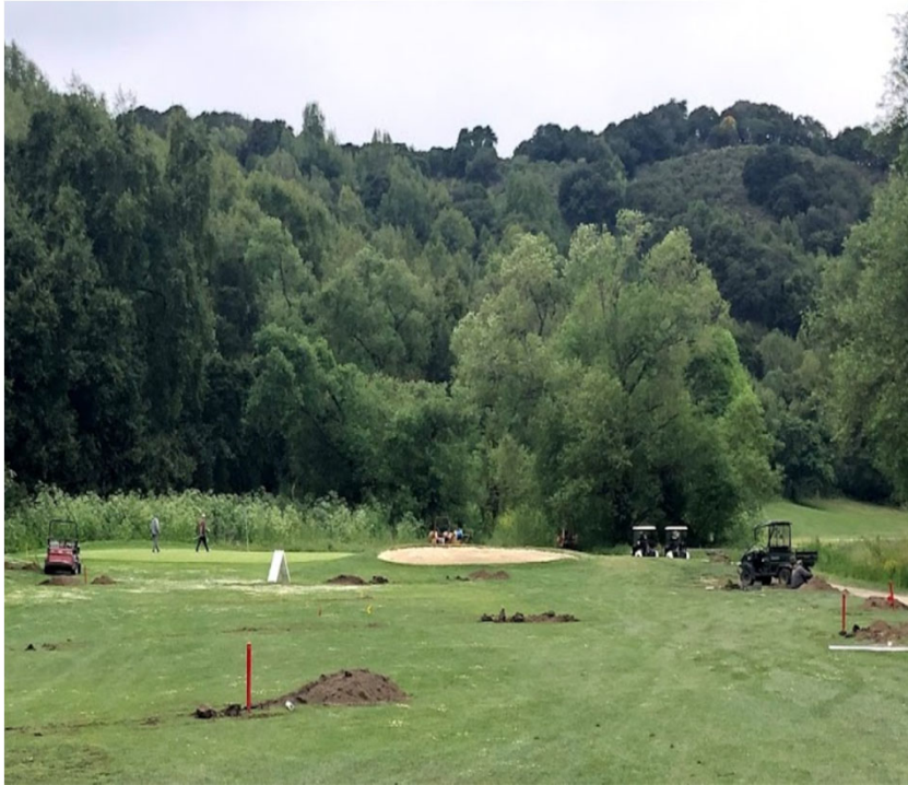
1 st hole Installation During COVID-19 Closure
